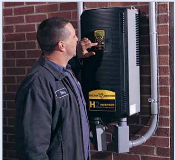
Baldor's VS1SP260-1B 60 HP adjustable speed drive was selected for a history of consistent performance and because it is simple to program and easy to operate.
